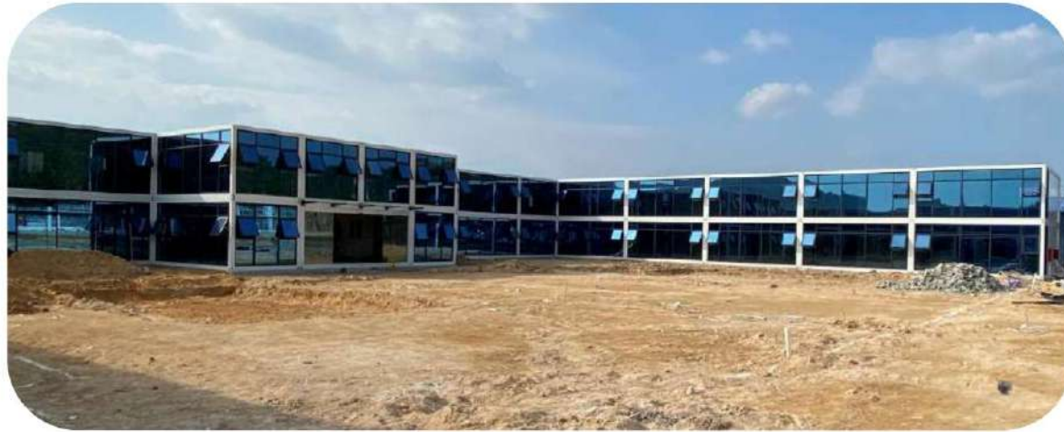
Horizontal + vertical multiple combination container Supporting concealed frame glass curtain wall
